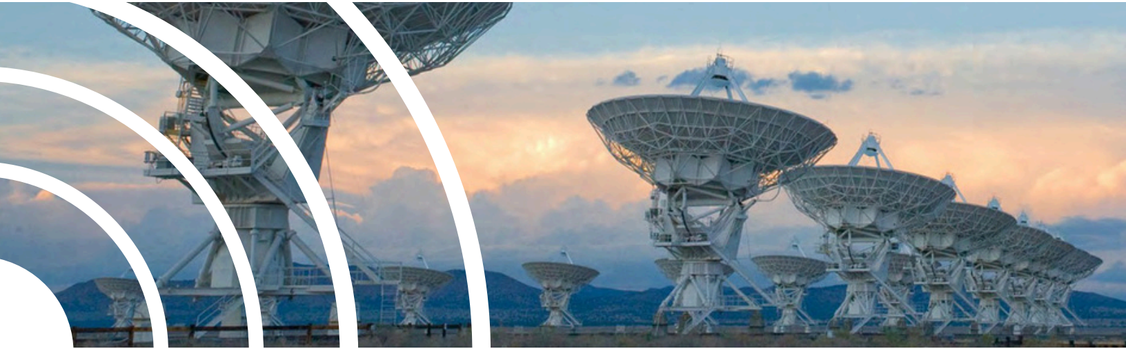
The Very Large Array (VLA) is a collection of 27 radio antennas located at the NRAO site in Socorro, New Mexico. Each antenna in the array measures 25 meters (82 feet) in diameter and weighs about 230 tons. Credit: Alex Savello/NRAO.
